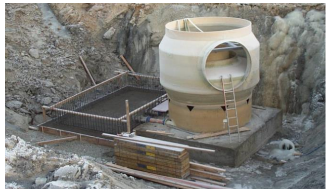
Figur 13 FluidSep under montering
