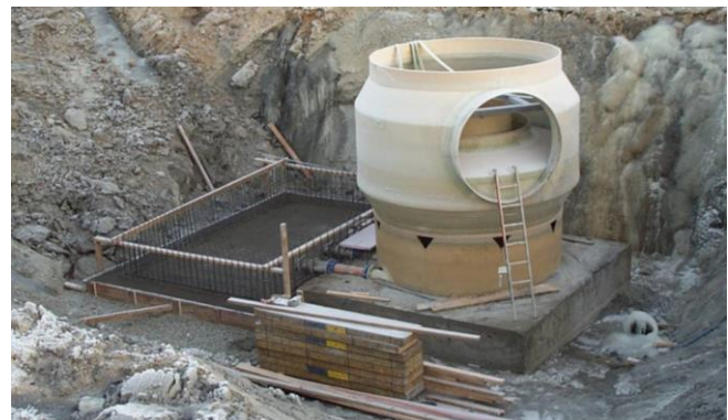
Figur 13 FluidSep under montering
